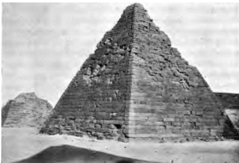
A PYRAMID AT GEBEL BARKAL, SHOWING THE ARRANGEMENT OF THE STONES AT ONE CORNER.
