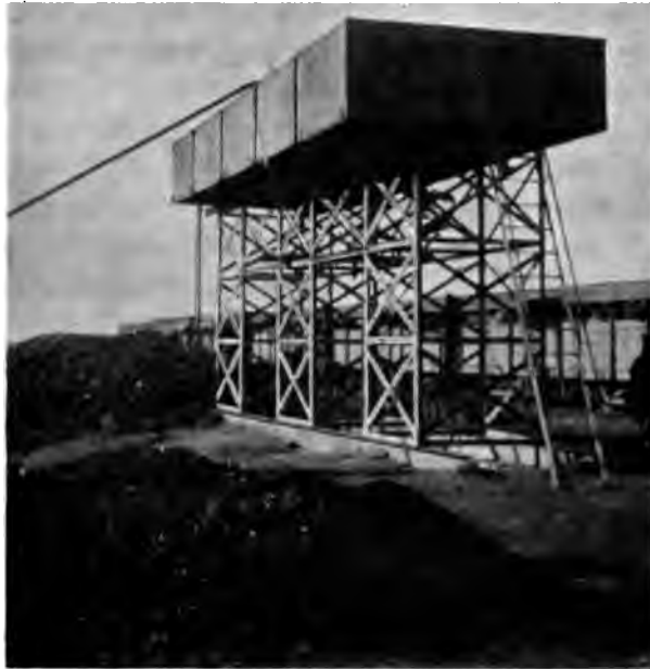
WATERING TANK AT NO. 6 STATION IN THE ABŪ-HAMED DESERT.
