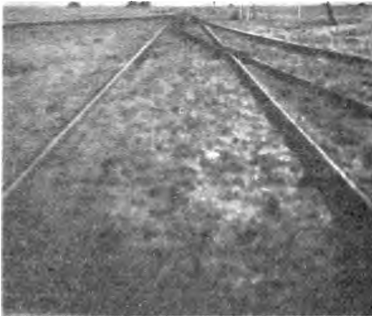
VIEW OF THE EXTENSION AT NO. 6 STATION IN THE ALABAMA DESERT.
